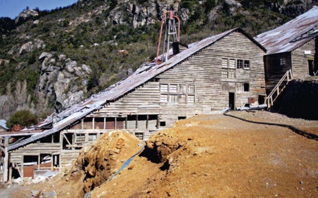
Fachada lateral Planta de Concentrado | Concentrating Plant side facade
